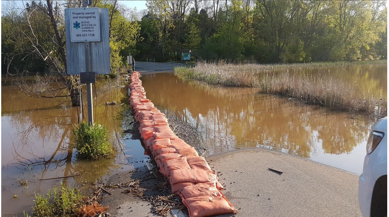
Figure 17. Record high lake levels and emergency barrier additions at the Cootes Paradise Fishway (above), and at Grindstone Marsh's Sunfish Pond area. The road to the Fishway has since been raised.
