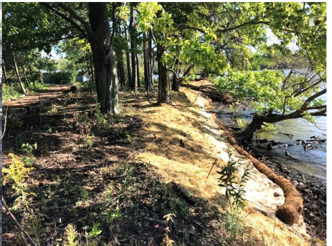
Figure 22. Shoreline reconstructed at outer Grindstone Marsh restoration site, May 2016 & July 2017 (above), and bioengineering repair of formerly eroded and undercut shore at Princess Point and near the RBG boathouse 2020 (lower).
