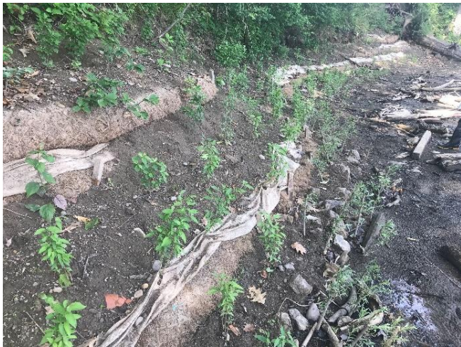
Figure 22. Shoreline reconstructed at outer Grindstone Marsh restoration site, May 2016 & July 2017 (above), and bioengineering repair of formerly eroded and undercut shore at Princess Point and near the RBG boathouse 2020 (lower).
