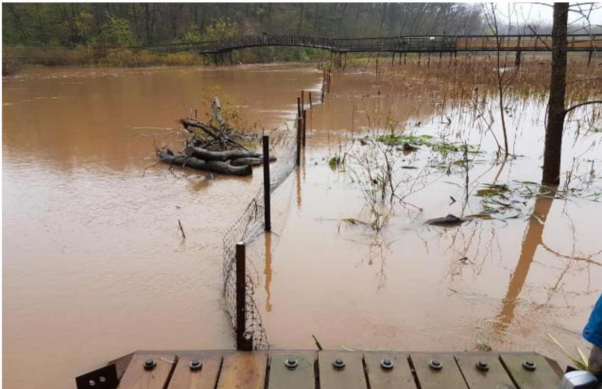
Figure 18. 2021 repair of Hendrie Valley carp exclusion berm by the pond 2 area (above), and 2019 emergency system with temporary fence in place during record high water levels (below).
