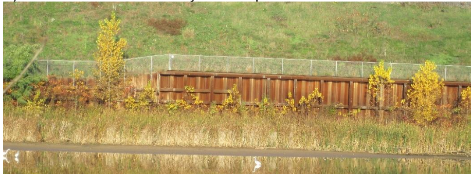
c) Sunfish Pond slope after shoreline stabilization plantings filled out.
