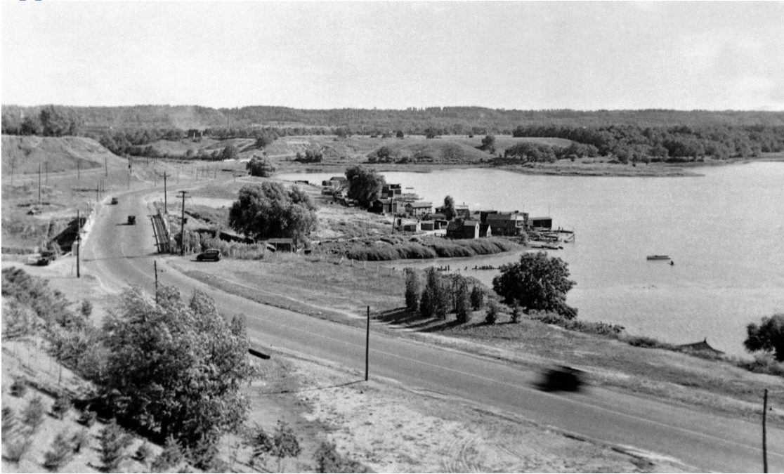
Figure I. Photo from 1935 taken from the Iroquois Bar (now Burlington Heights) facing southward towards Princess Point; notice that the Princess Point peninsula elevation appears to be level with the area that is now termed lower Prairie, thus this photo was taken before fill had been dumped and leveled on top of the peninsula
