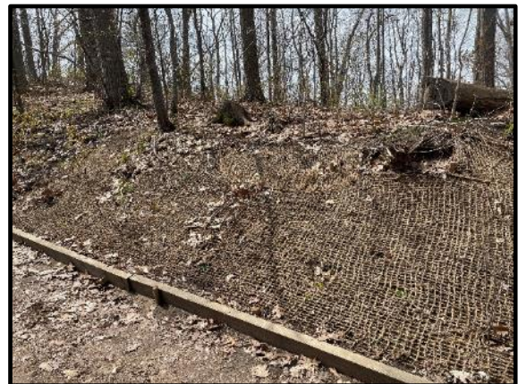
Before slope stabilization (left) and after coco fibre net installation and native plant restoration work (right).
