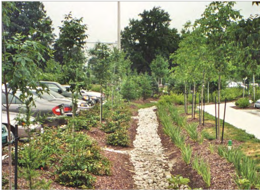
Example of a vegetated filter strip
