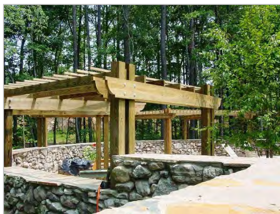
Example of a shade structure
