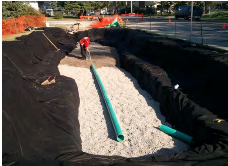
Example of a rain garden construction
