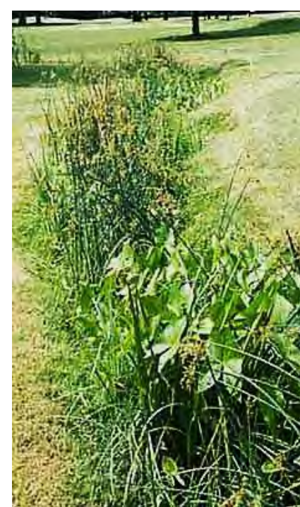
Example of a swale
